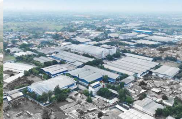
Tangerang Plant, Indonesia (Filtration & Other Products)
